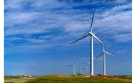
Wind towers in Codrington, Victoria
