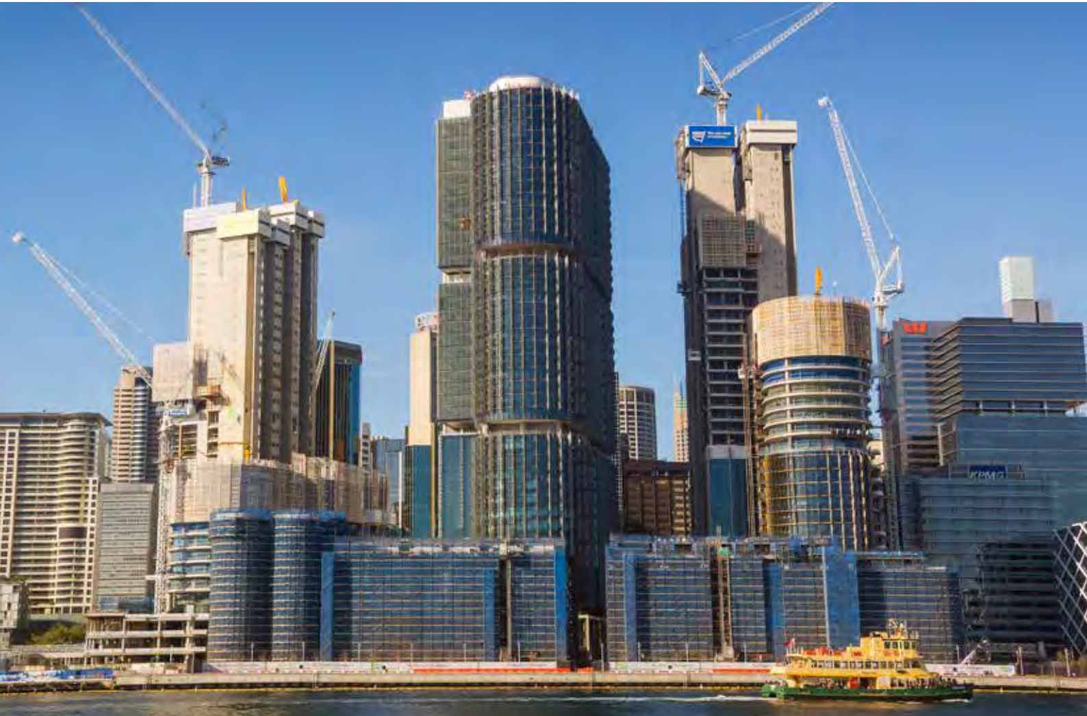
The Barangaroo Delivery Authority intends for Barangaroo to become carbon neutral
