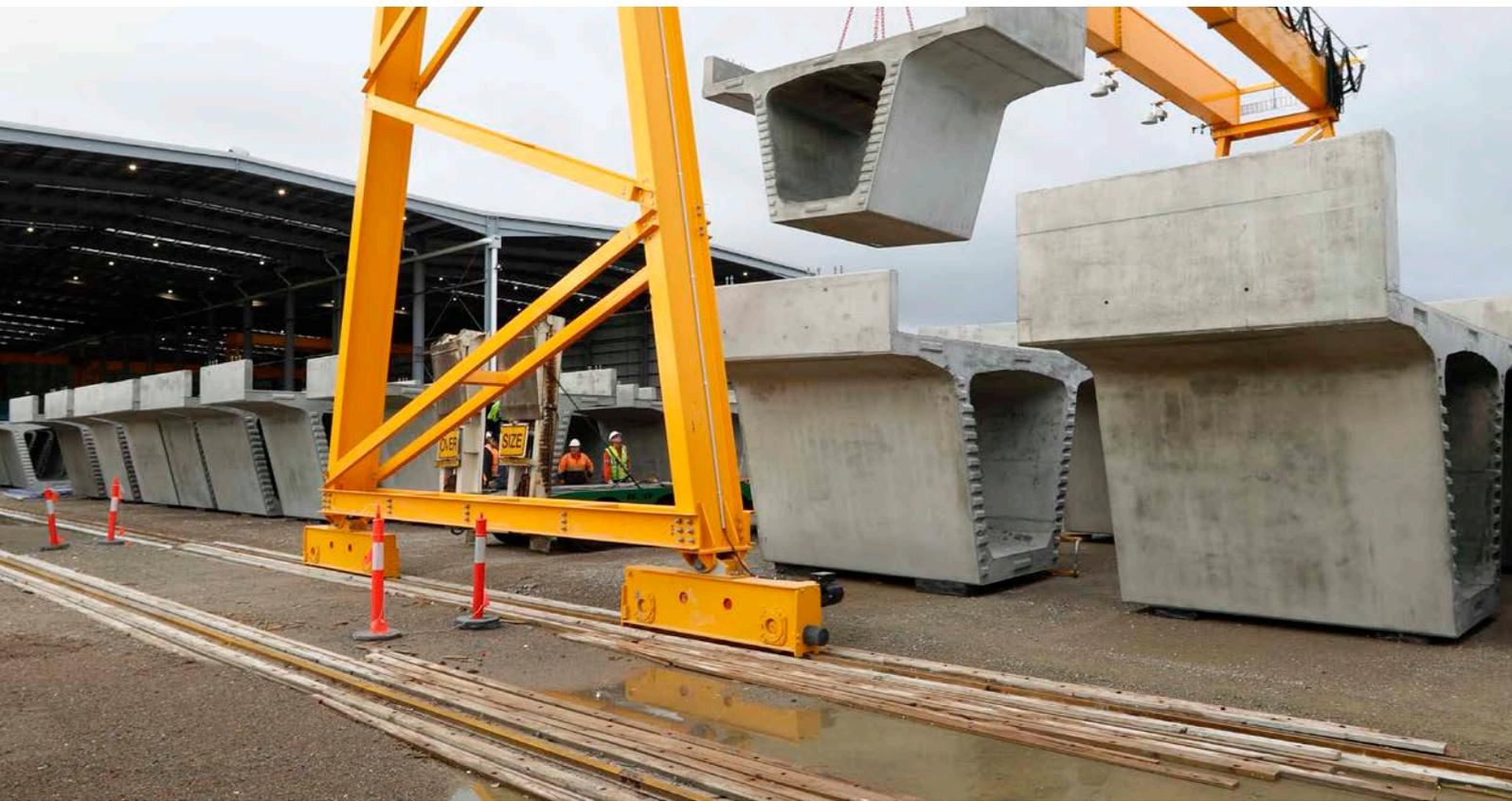
*Diesel powered gantry crane in action lifting a 26-tonne concrete segment.*
