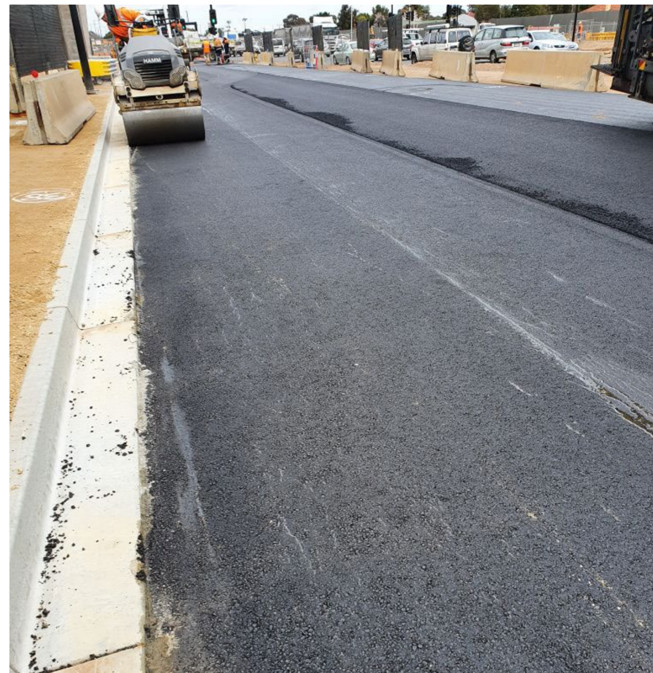
Reconophalt™ 100% recycled asphalt on the Regency Road to Pym project
