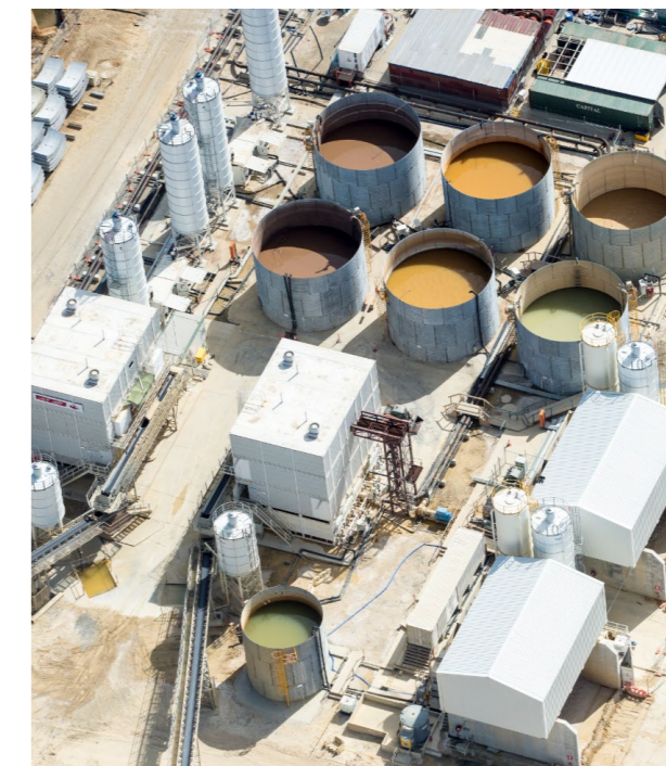
Slurry treatment plant at High Wycombe supporting tunnel boring
