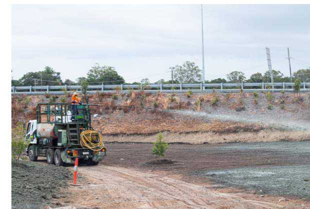
VE Gro-Matt being applied at the CR2SM project in Queensland
