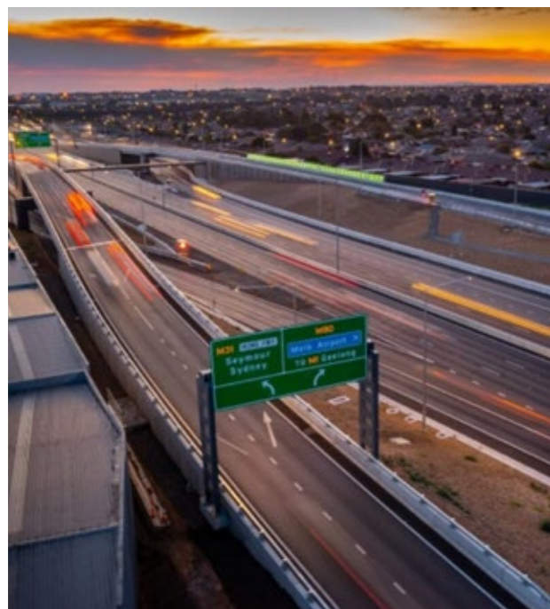
M80 Upgrade (Sydney Road to Edgars Road), Victoria, CPB Contractors - awarded the 2023 Australian Construction Achievement Award (ACAA).
