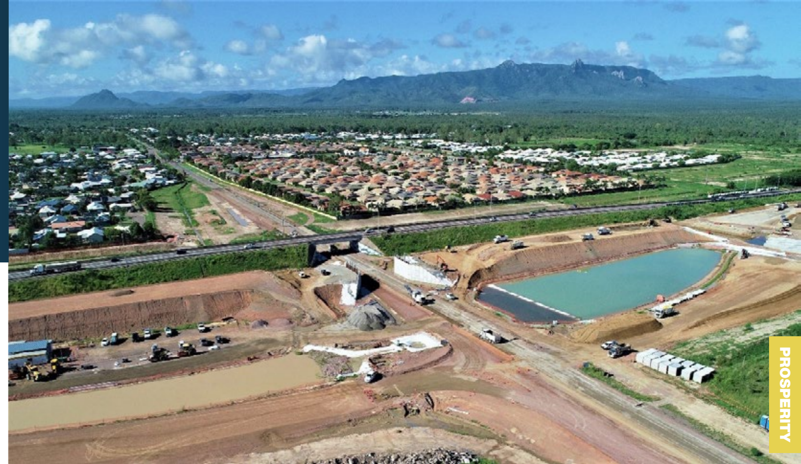
Beck Drive Interchange HES Basin February 2022 – Image Courtesy Georgiou Group
