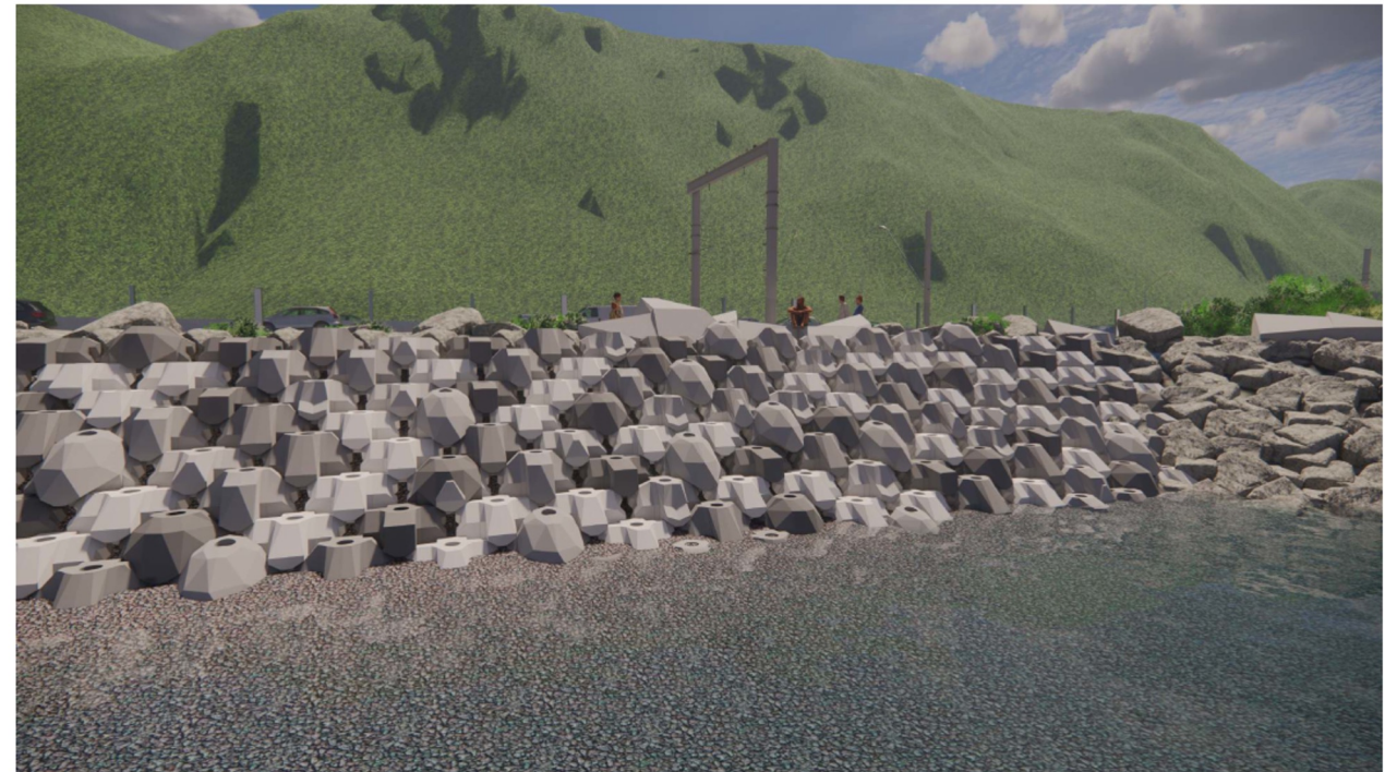
Macro Value Opportunities—Coastal Revetment. Concrete Block Revetment Optioneering. Te Ara Tupua Alliance.
